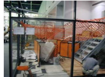
Figure 1: The Orange Arena
